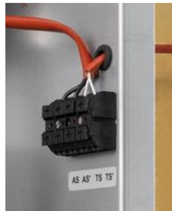
Figure 35 terminal for auxiliary contact connection
