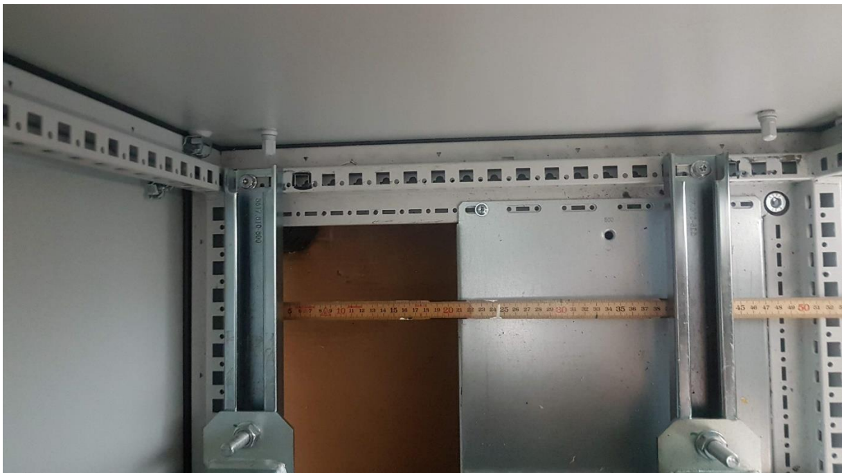
Figure 7 opening at the bottom of the cabinet (top view from inside). About 1/3 remain open.
